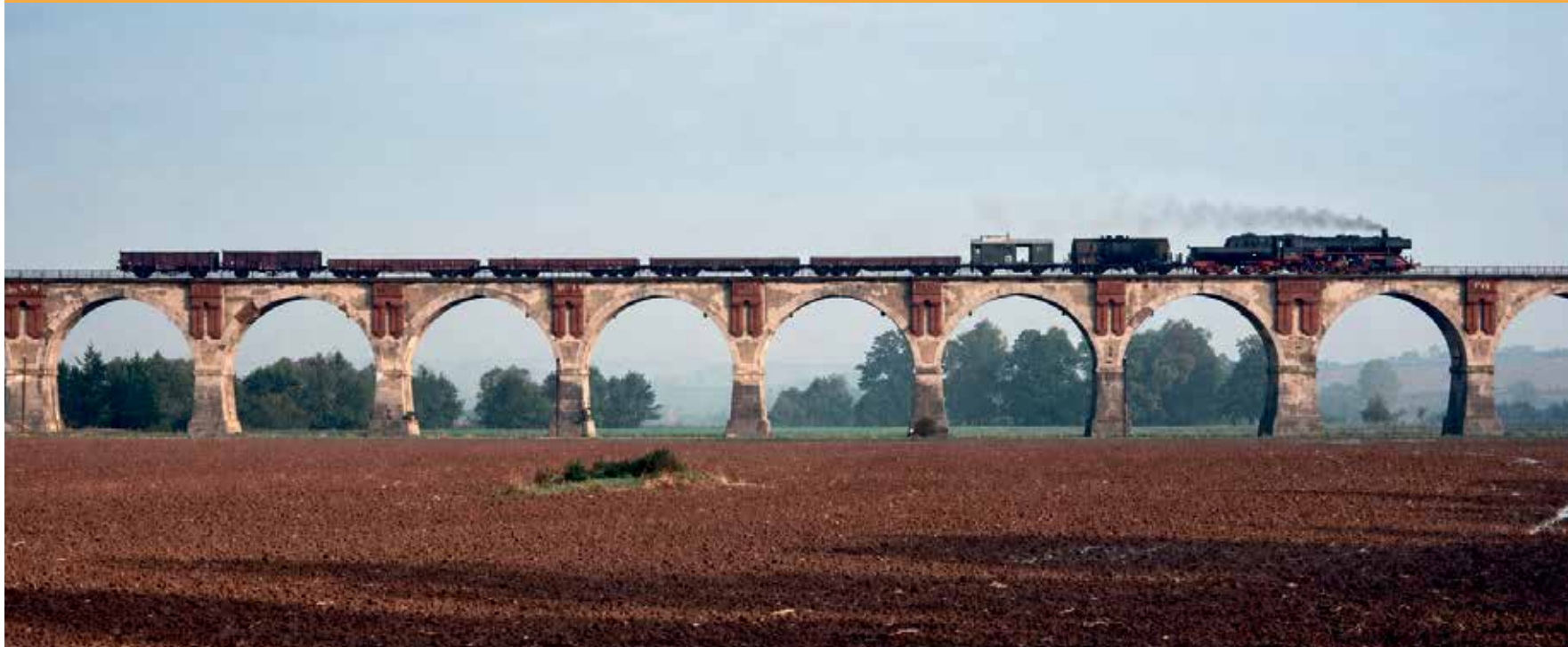
Viadukt in Frohnsdorf.
